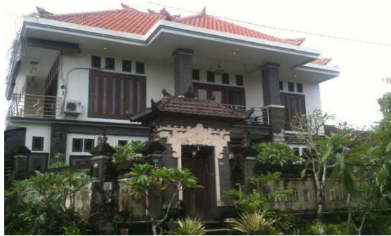
Figure 4 Kontemporer dwelling without traditional Balinese ornaments but adopting penyengker / fence and angkul-angkul Source: rumahin.wordpress.com
