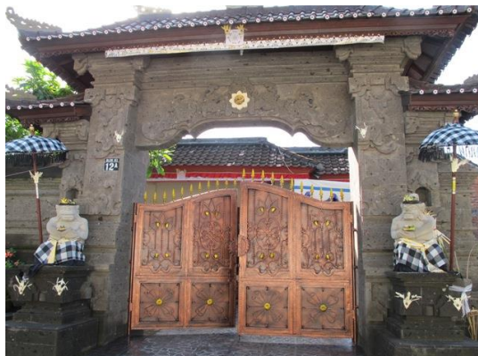
Figure 3 Widened angkul-angkul Source: https://1219251059ninyomanlitanugrahenidewi.wordpress.com
