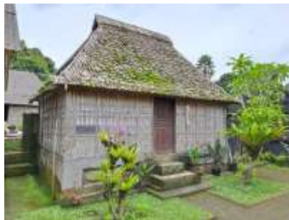
Figure 2. Paon as one the Architecture Building which should not be removed Source: Arta, 2022
