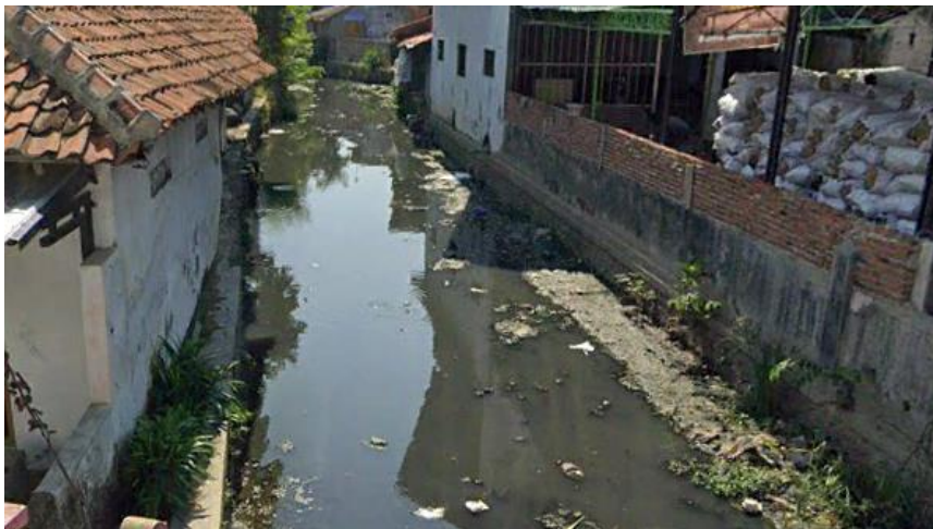
Figure 2. Sedimentation on Jembangan River Source : google earth street view
